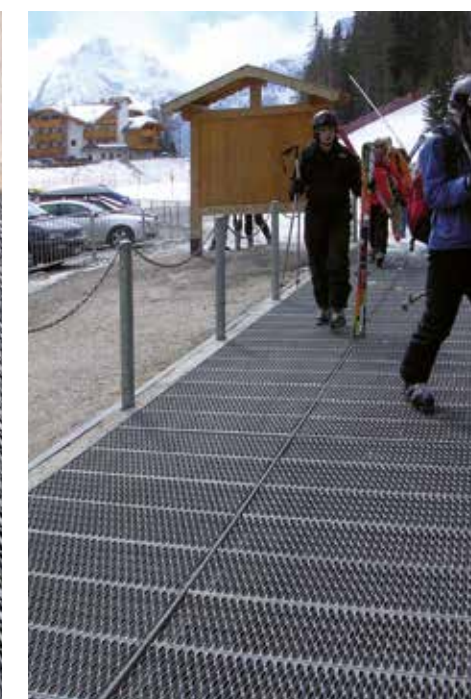
Canazei: camminamento antiscivolo tipo Graepel Gripp, ingresso cabinovia Canazei: anti slip walkway made of hot-dip galvanized Graepel Gripp, front of the entrance of a cableway
