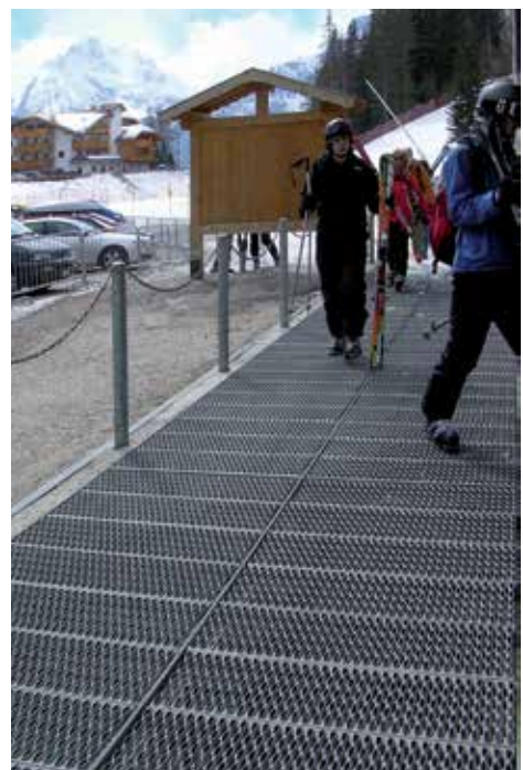
Canazei: camminamento antiscivolo tipo Gripp, Ingresso cabinovia Canazei: anti slip walkway made of hot-galvanized Graepel Gripp, front of the entrance of a cableway
